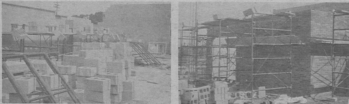
Construction progress on Clio Lodge new Masonic Temple
